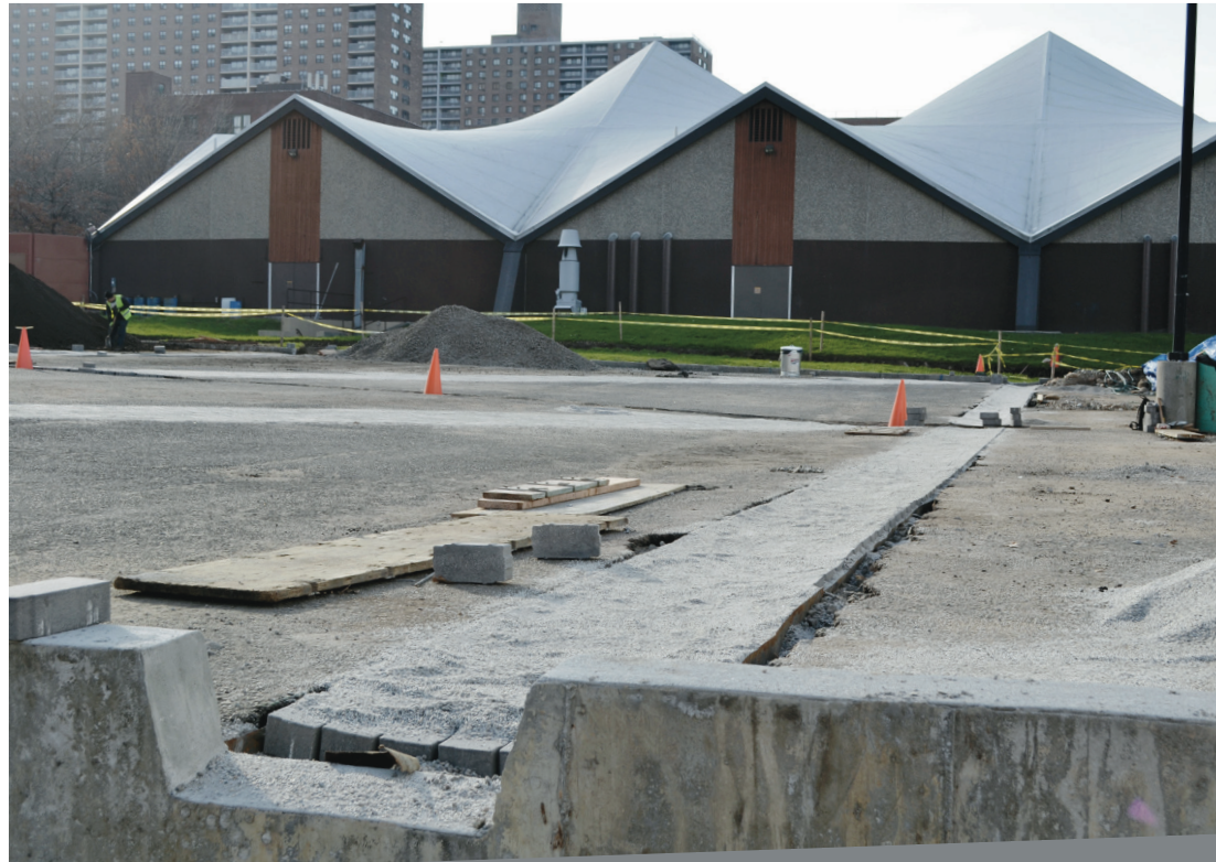
Condition during the construction process
