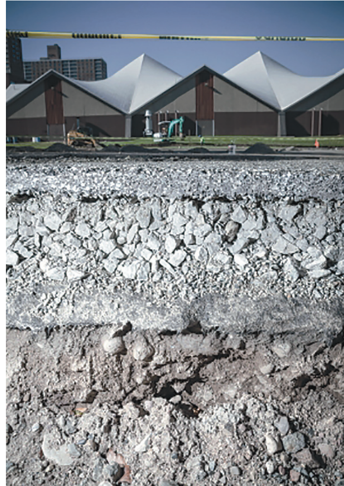
Sub-surface section, prior to intervention
